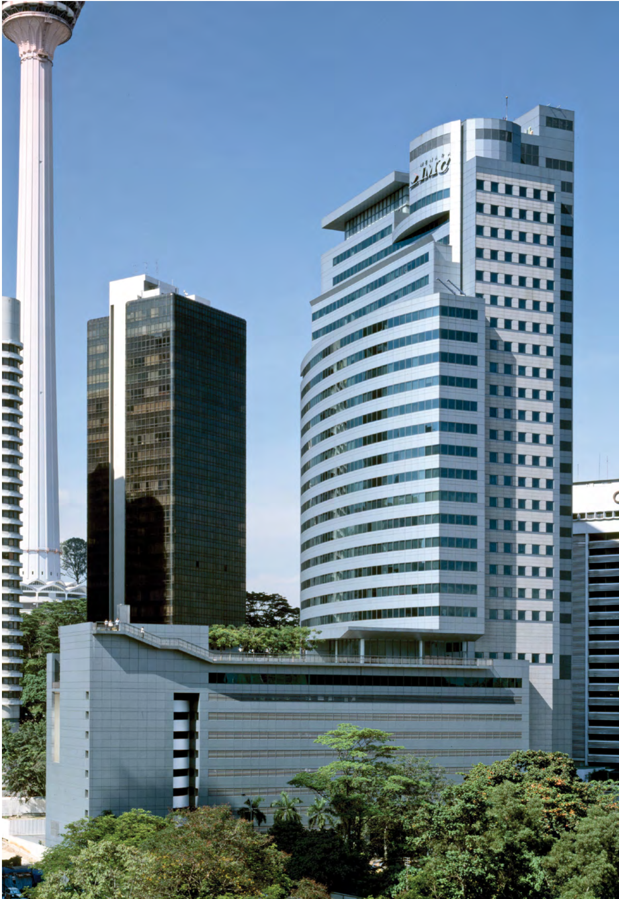
Tsao And Mckown, IMC Building, Kuala Lumpur, 1996
