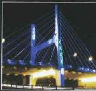
Tabriz Cable Stayed Bridge
