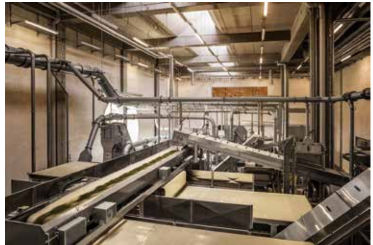
[Retrieved September 28, 2016 From http://www.archdaily.com/634724/ricola-krauterzentrum-herzog-and-de-meuron ]
