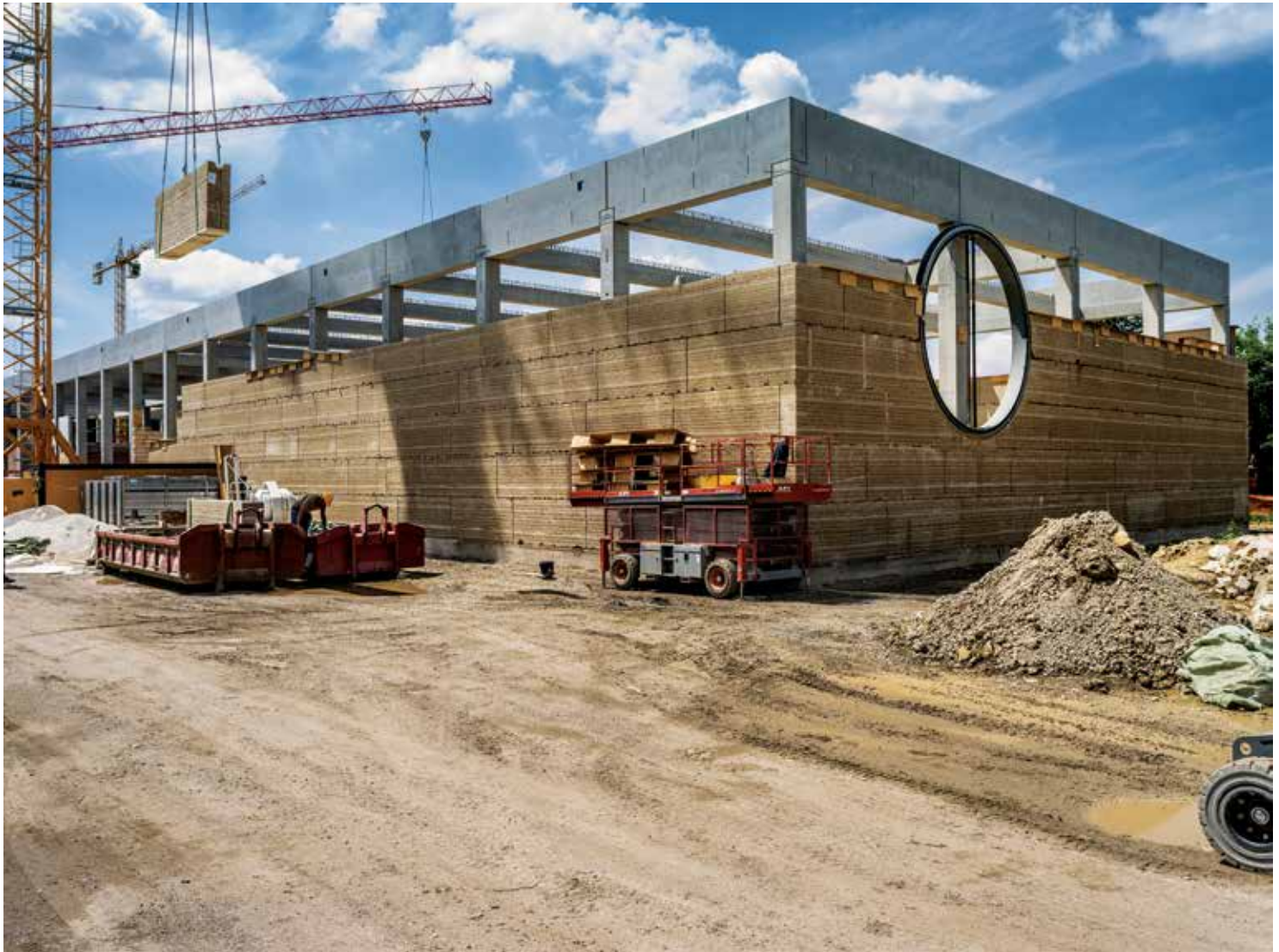
[Retrieved September 28, 2016 From http://www.archdaily.com/634724/ricola-krauterzentrum-herzog-and-de-meuron ]
